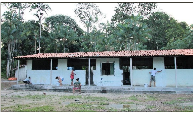
Alegre Vamos School in need of paint and repair
