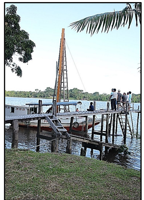
Barge drives down 37-ft posts for docking medical boat at Paritá
