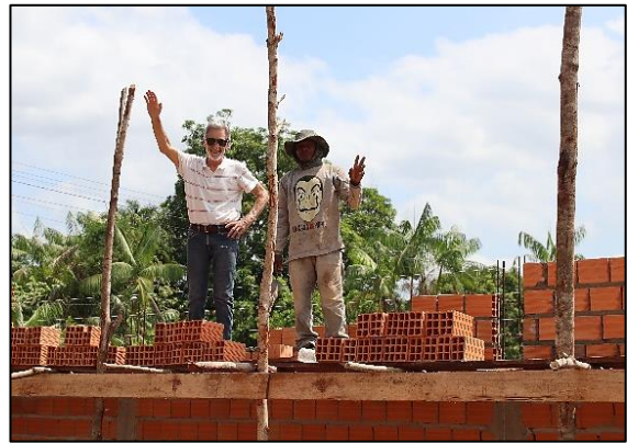
Scott with Vila Aviva builder on wall going up around property
