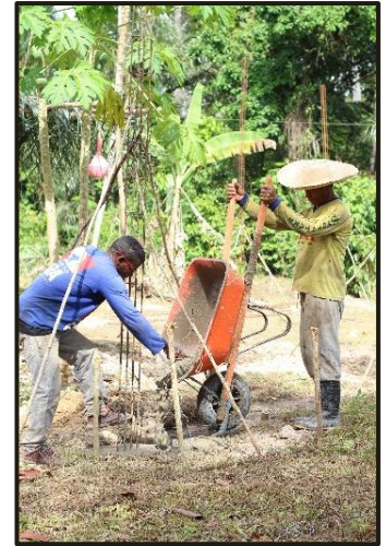
Right - Pouring concrete foundation
