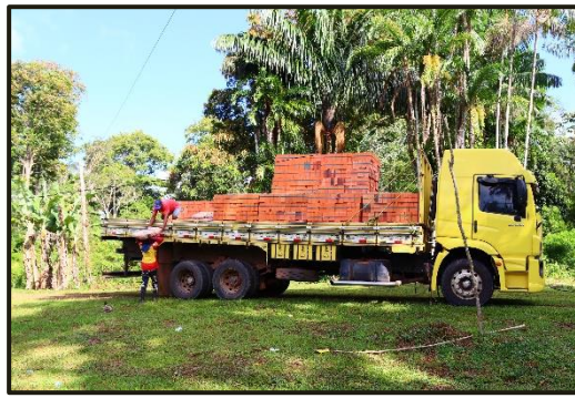
Truck load of bricks and cement arrives
