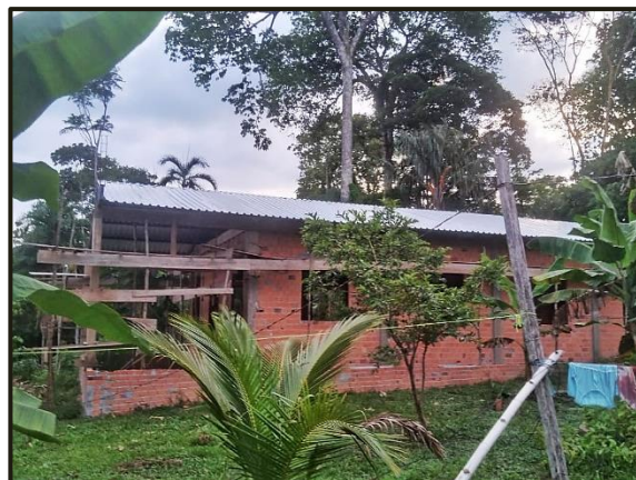
Side view of Alegre Vamos church with zinc roof installed
